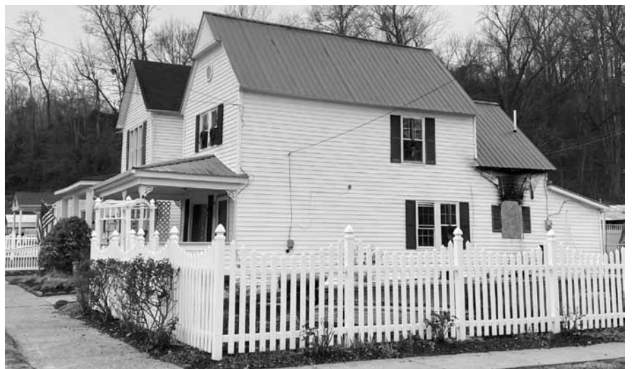
Fire damage at Delcie's House.
